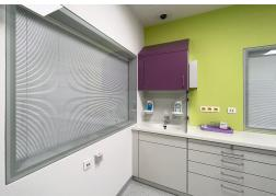
With the system of partition panels, a glazed window panel represents one of the basic elements to construct clean workplaces and areas with maximum safety, sterility, hygiene, easy maintenance and sanitation.
