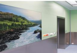
The graphic panel is a state-of-the-art design solution, a part of the partition system for the construction of clean rooms and workplaces with the maximum sterility, hygiene, easy maintenance and sanitation.
