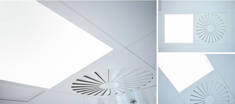
LED fixtures are used for the lighting of interiors with basic environment. They are mostly flushmounted in the lightweight metal suspended ceiling /LP/ For Clean, a.s. The light fixture features IP 44 ingress protection from the top and IP 54 ingress protection from the bottom according to EN 60529 (IEC 529).
