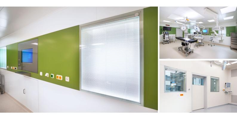
With the Surgical system, a glazed window panel represents one of the basic elements for the construction of operating theatres with maximum safety, sterility, hygiene, easy maintenance and sanitation.
