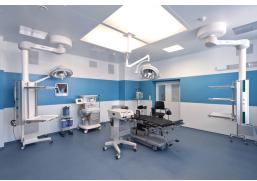
The laminar flow field for operating room are used to create a uniform airflow of specific cleanliness in septic and aseptic operating theatres.
